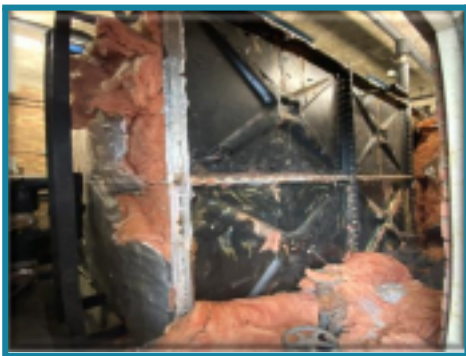
Before and after - Trove Court water tank replacements
